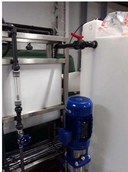
Representative image skid connections of flushing in the same frame.
