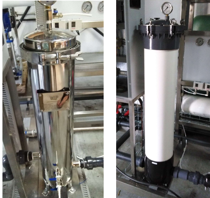
Optional. Multi-cartridge filter image in stainless steel and PVC respectively.
